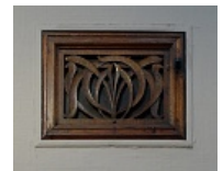
Fretwork cover of ventilation duct
