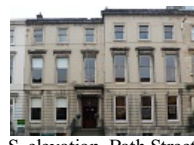
S. elevation, Bath Street
