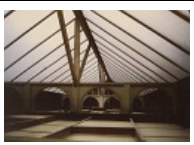
Roof glazing looking W.
